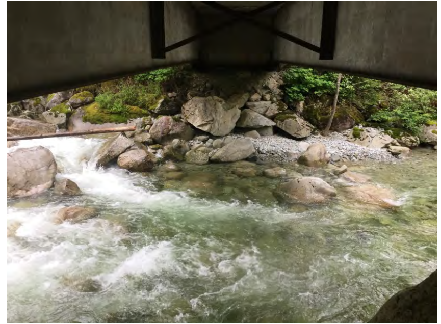
Left Bank Abutment when facing downstream
