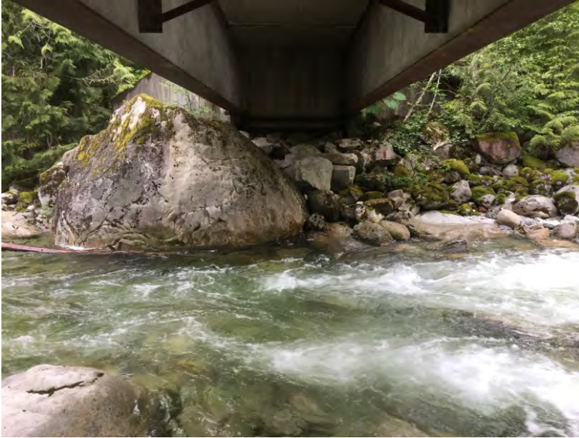
Right Bank Abutment when facing downstream
